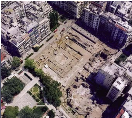
VIEW OF THE SITE FROM THE SOUTHWEST. PRE-INTERVENTION (1996).
